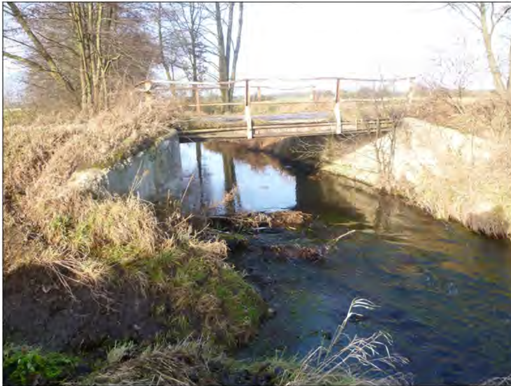
Abb.4: Salzwedeler Dumme Brücke, Station 12+588
